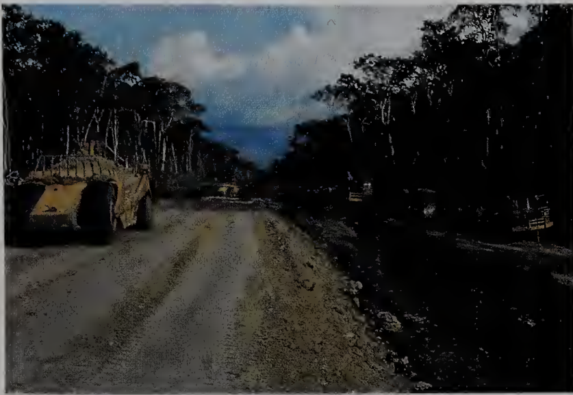
FIGURE 27.13 The Trans–Amazon Highway in construction cuts a great swath through the rainforest and requires extensive earth moving to grade the roadbed and provide drainage. (Toby Molenaar/Woodfin Camp.)
