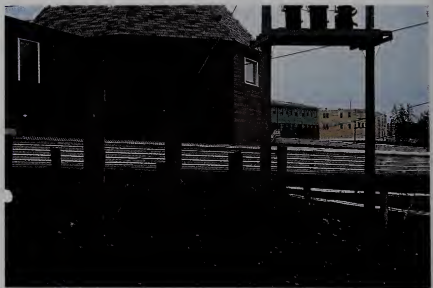
FIGURE 15.38 The elevated tunnel of sheet metal is a “utilidor” (utility corridor) in which steam and water lines are protected from freezing in the severe tundra winter. Notice that the buildings are mounted on posts and have small windows. Inuvik, Northwest Territories. (Mark A. Melton.)
