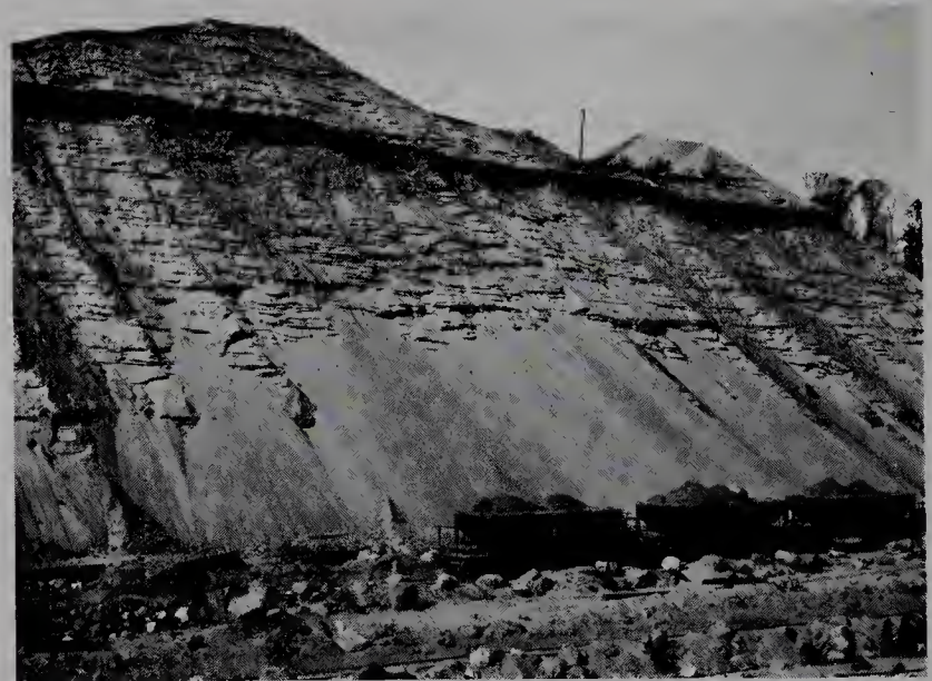
FIGURE 22.32 Thick layers of outwash sands and gravels such as these on the north shore of Long Island were excavated in great quantities for use in highway and building construction. The dark layer at the top is a bed of glacial till left by a glacial advance. Boulders in the foreground are glacial erratics that have rolled down from the till bed. Exposures such as this are rarely seen today in this region. (A. K. Lobeck.)
