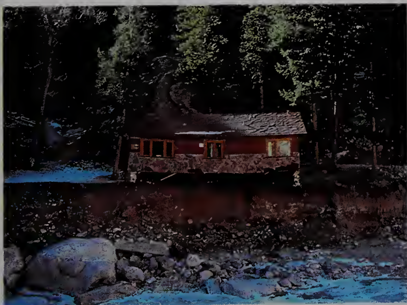
FIGURE 17.8 Rapid bank caving undermined this cabin on Big Thomson Creek, Colorado, during a disastrous summer flood in 1976. Alluvium was flushed out from the channel floor in the foreground leaving only scoured bedrock and a litter of large boulders. (David C. Shelton, Colorado Geological Survey.)
