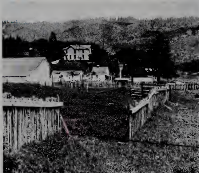
FIGURE 14.28 During the San Francisco earthquake of 1906, this fence was offset 2.4 m (8 ft) by lateral movement along the San Andreas Fault near Woodville, California. (G. K. Gilbert, U.S. Geological Survey.)
